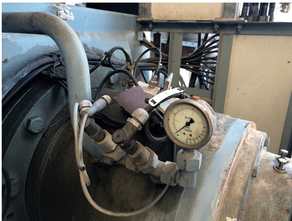
Figure 5-21 Shifting mounted components to check the measurement
