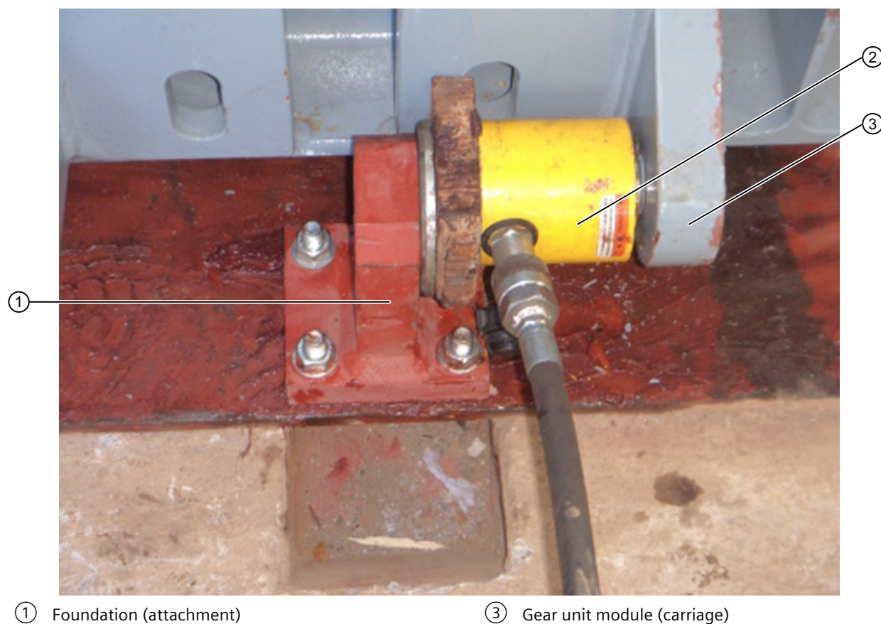
Figure 9-5 Alignment (displacement) of the gear unit module with the hydraulic jack
