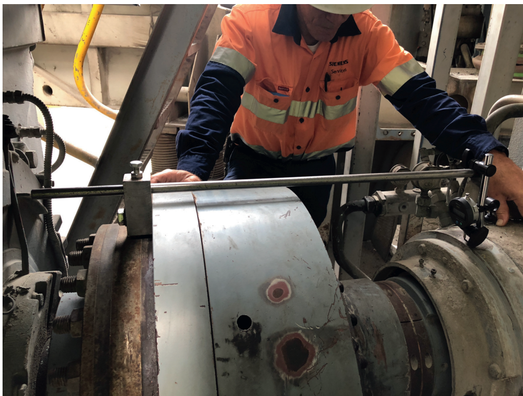
Figure 5-22 Turning the motor shaft by hand with mounted measuring equipment: The following diagram shows measuring the dimension "b1" (angular offset):
