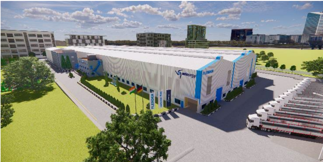
The Flender location in Chennai with two, new production halls on the right.
